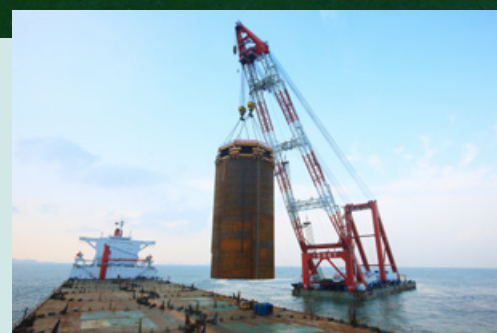
Zhenfu No. 8 of ZPMC lifting steel cylinders.
